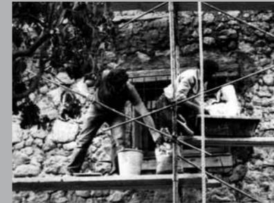
*Before building the walls, as many local materials as possible are collected : limestone, sandstone, tufa as well as pebbles from the local river. Mortar is obtained by mixing binder lime or plaster, with sand and water. The lime is made by heating limestone in a kiln, which is then crushed. The plaster is made by heating and crushing the « plasterstone », the gypsum.*
